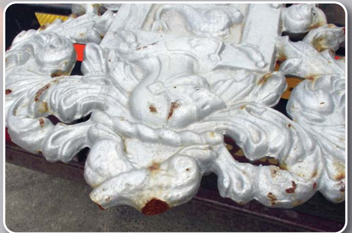
Each of the castings was assessed for damage and subsequently repaired at our workshops.
