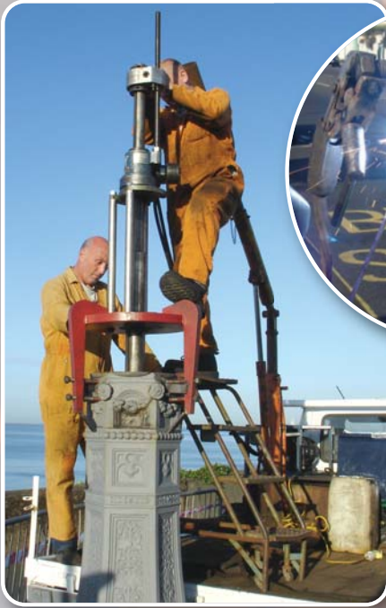
The column spigots were built up with gas fusion weld, and along with the mounting face, re-machined. The finished castings were then returned to site.
