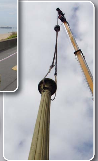
The column is lifted into position and the spigot is dropped into the base.
