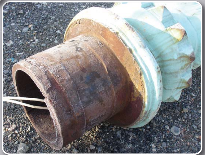
Spigots that locate the columns into the base's were worn, allowing the the lamps to rock dangerously.
