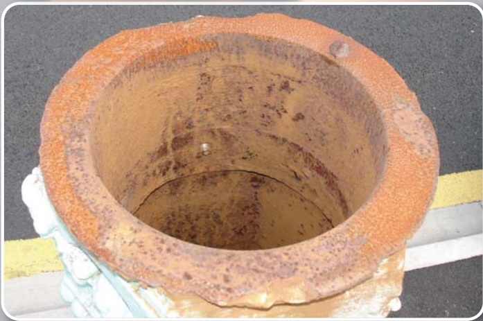
The base which receives the column is eroded and will require reaming out to accept the rebuilt and machined spigot.
