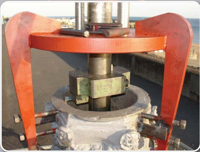
The reaming tool gets to work.
