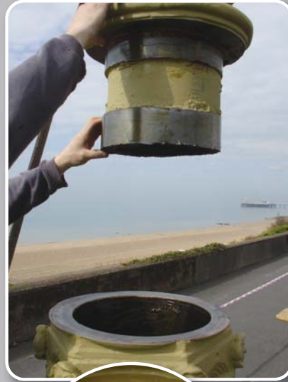
The column is lifted into position and the spigot is dropped into the base.
