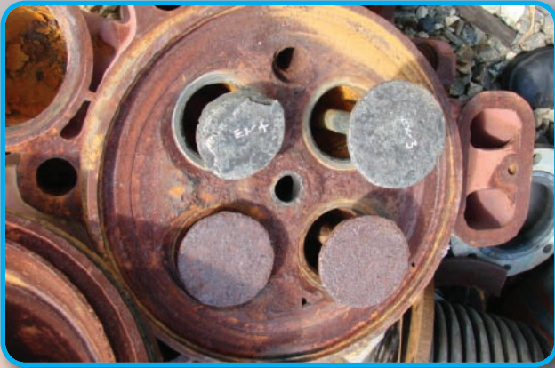
Excessive rust or corrosion on interior or machined faces
