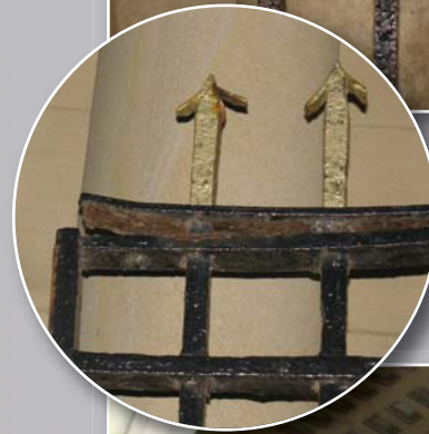
The collision has distorted the metalwork, loosening the leaded joints.
