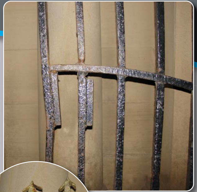
The collision has distorted the metalwork, loosening the leaded joints.
