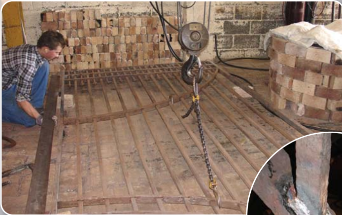
The gates were cleaned of built-up paint layers, jigged up and straightened out.
