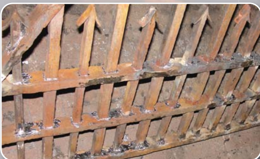
The gates were cleaned of built-up paint layers, jigged up and straightened out.
