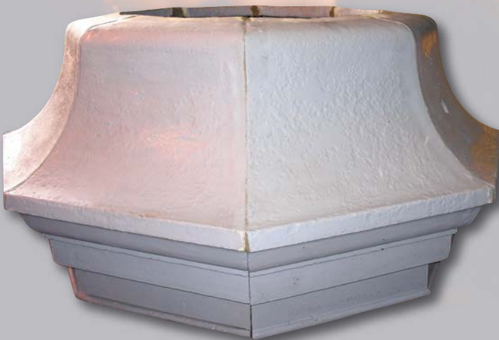
The restored segments are primed and bolted together ready for transport back to Moseley Road.
