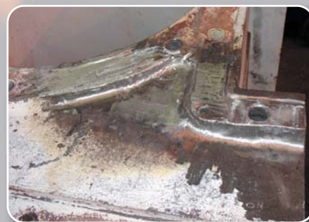
Welded area dressed to original profile ready for re-machining.
