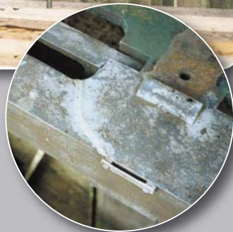
The underside of the bridge showing the scaffolding in place ready for the removal of the sluice gate mechanism. A poorly executed third-party arc weld showing extensive cracking.
