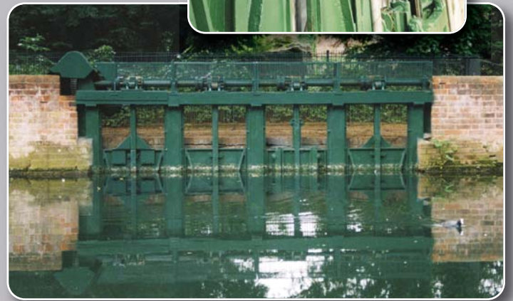
Completed sluice gates with restored mechanism and guards.
